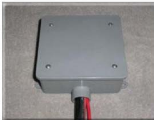
Energized outlet: outlet box with cover and electrical receptacle (6-50R)
